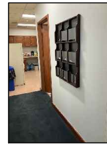
B. Wall to be removed.
