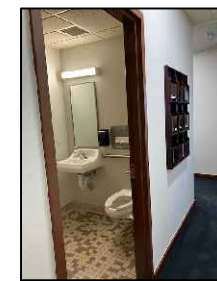
C. Door and frame to be removed.
