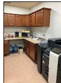
G. Flooring to be replaced.
