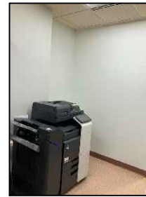
A. Wall to be removed.
