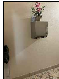
G. Toilet accessories to be removed.
