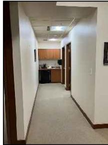
B. Carpet removed up to office door.
