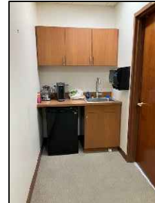
C. Existing cabinetry, counter and paper towel holder removed.
