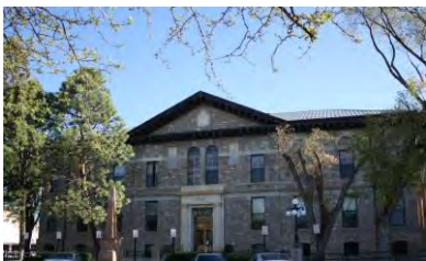
Santiago E. Campos Courthouse, Santa Fe
