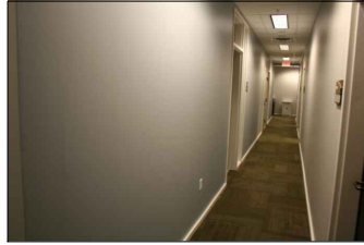
D. Hallway 296 - East
