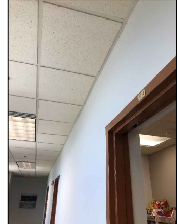
G. Bulkhead for ceiling grid.
