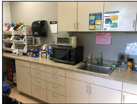
B. Cabinetry to be replaced.
